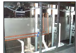
6) Install plumbing, electrical and soda lines.
